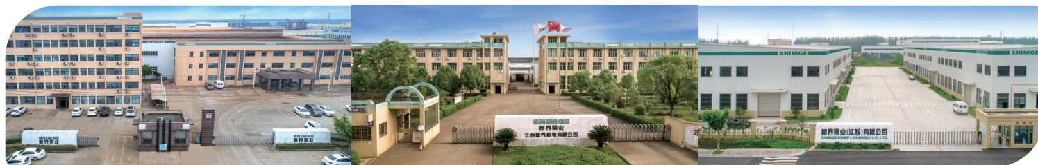
Shimge's casting parts production base in JiangSu Province
